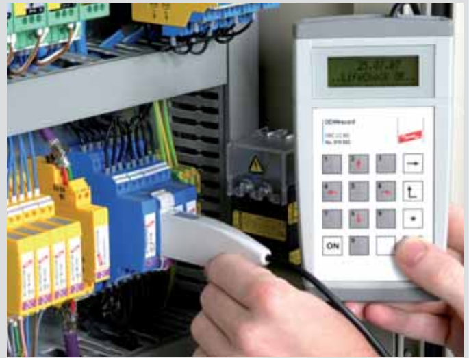
Testing an SPD module with RFID technology (LifeCheck)
