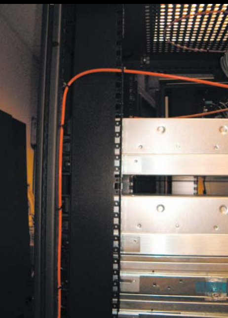
The red Firetrace Detection Tubing can be located in the rack in a manner that does not interfere with installation or maintenance of the equipment.
